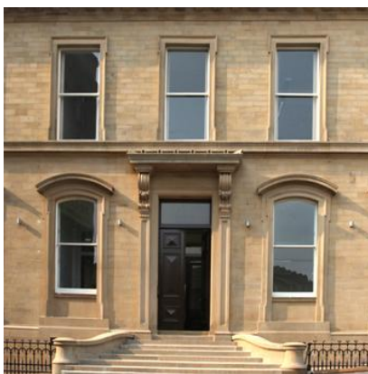
Shaw Lodge House (refurbished)
