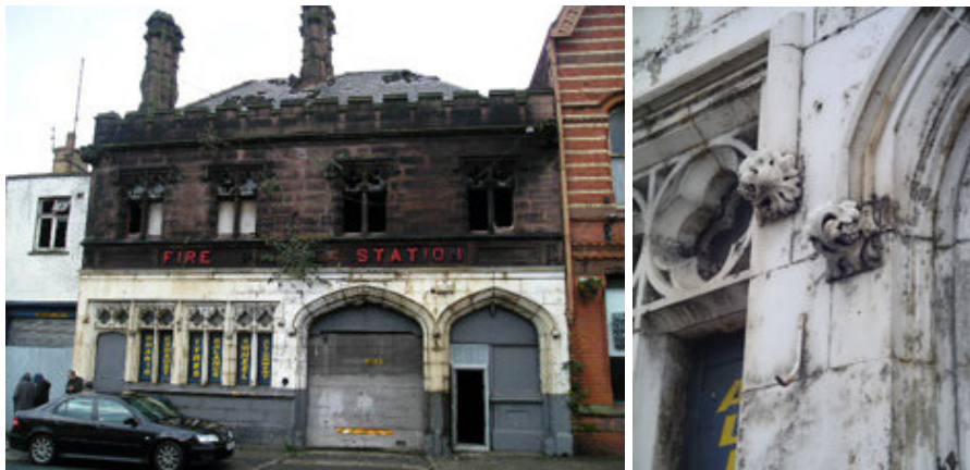
Front elevation of Fire Station, and architectural detail
