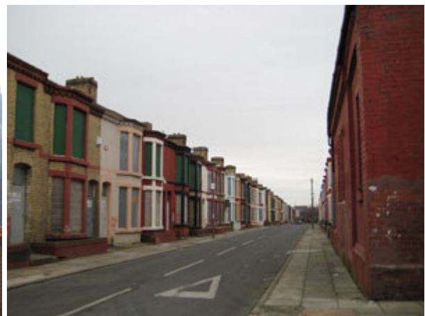
Boarded up houses down Nuttall Street
